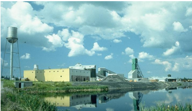
Surface buildings of an underground mine.
